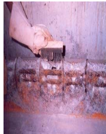
Fig 3: Removal of dust and rust
