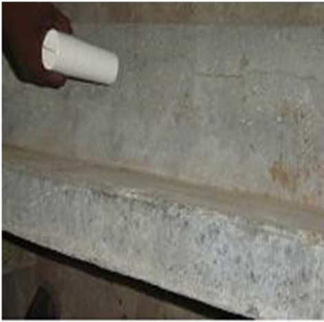
Fig 9: Roughening of GFRP laminates
