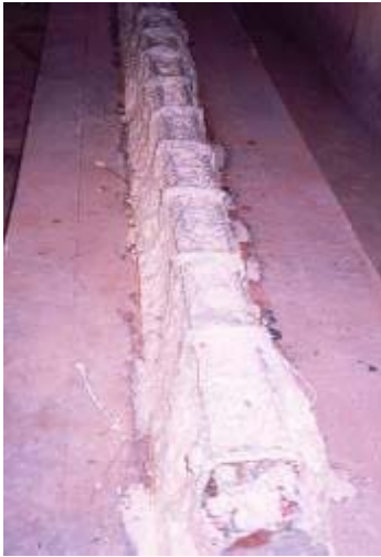
Fig 5: Application of bond coat
