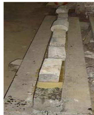
Fig 16: Application of weight
