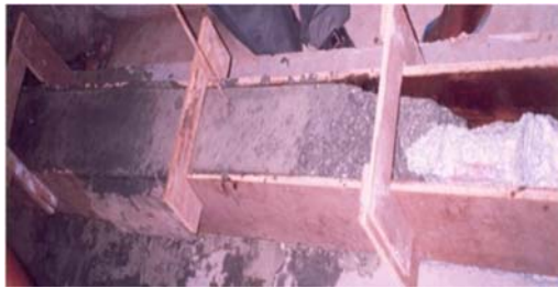
Fig 6: Application of polymer modified concrete
