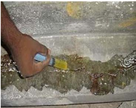
Fig 11: Sealing of cracks in web
