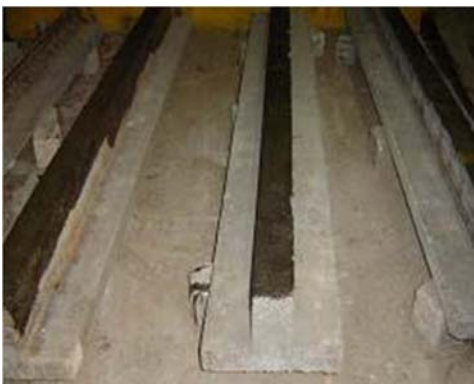
Fig 12: Sealing of cracks at soffit
