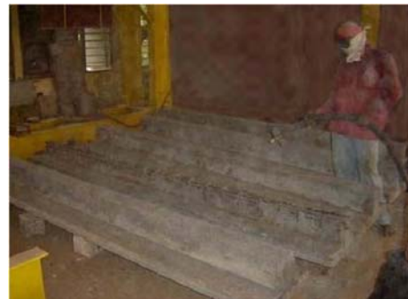
Fig 8: Sand blasting on tension face of damaged beams
