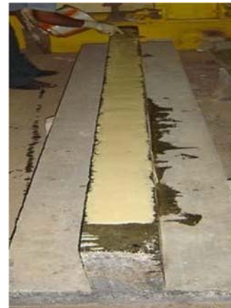
Fig 14: Application of adhesive
