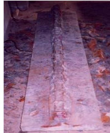
Fig 2: Removal of cover concrete
