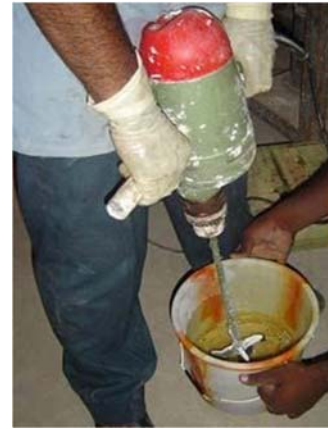
Fig 13: Mixing of adhesive
