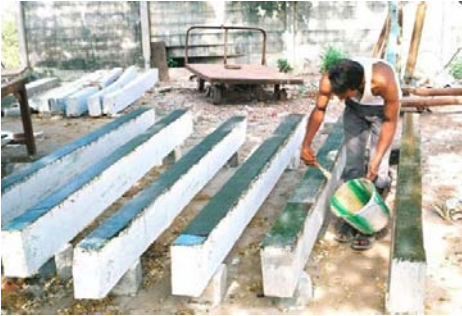
Fig 19: Finished With Protective Coating
