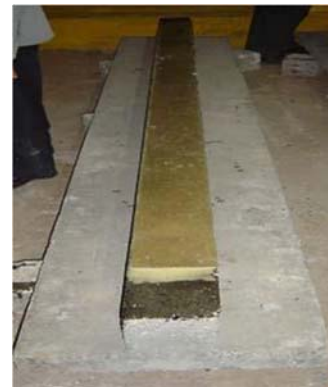
Fig 15: Fixing of GFRP laminates
