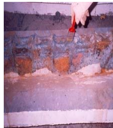
Fig 4: Anti-corrosive coating
