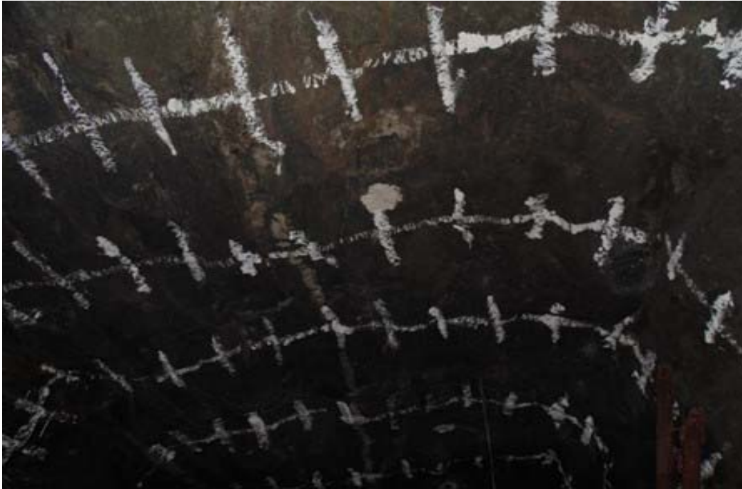
Fig 1: Properly marked rings
