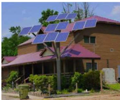
Fig 4: Mounting of Solar Tree near the house
