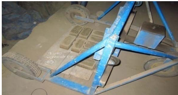
Fig 3.3: Casting of bricks
