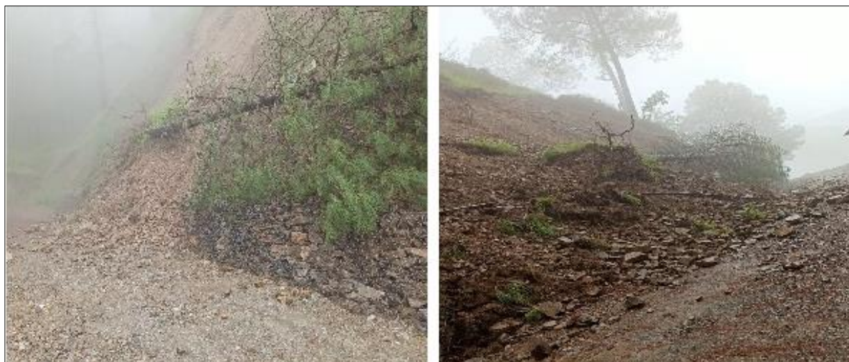
Plate 3: Landslide events along the road sides in the study area.
