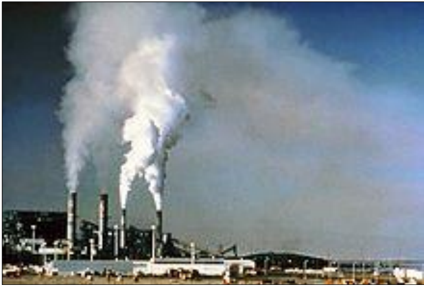
Fig 4: Before flue-gas desulfurization was installed, the air-polluting emissions from this power plant in New Mexico contained excessive amounts of sulfur dioxide.
